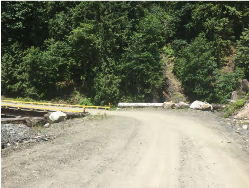
Approach from Left Bank when facing downstream
