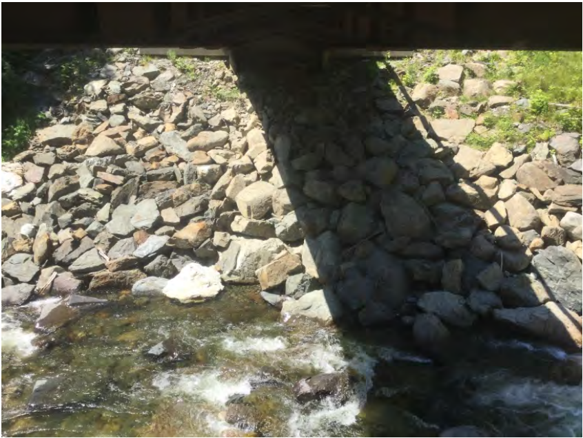
Right Bank Abutment when facing downstream
