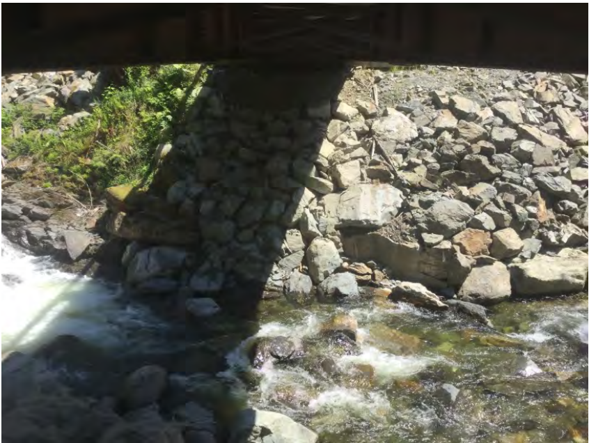
Left Bank Abutment when facing downstream
